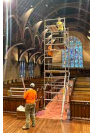
New energy-efficient LED lights and a digital dimming system are being installed in the church. Also pictured, rewiring the new dimmer system in the basement. The dimming project will be completed on March 11 when the system is programmed.
